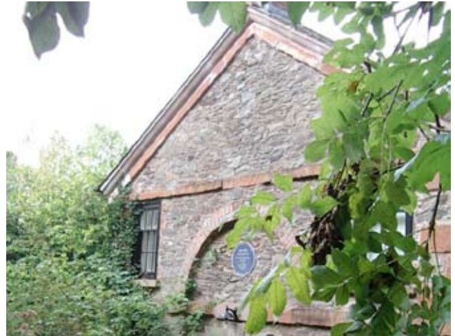
Fig 7. Drumbeg lock-keepers house
